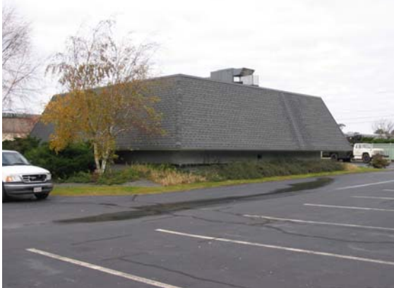
Wastewater treatment plant building
