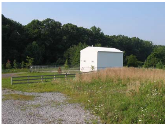
Wastewater treatment plant building
