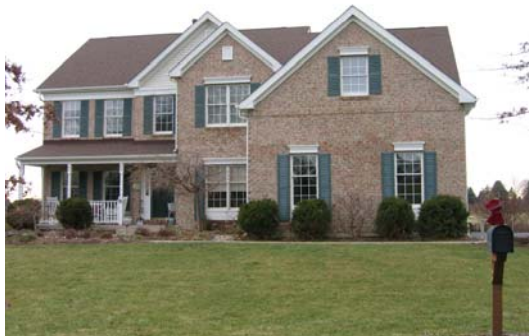
Typical home served by wastewater treatment facility
