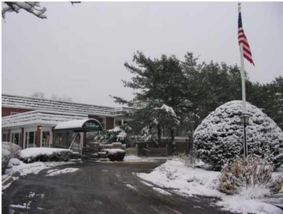
Entrance to Woodbriar-Atria facility
